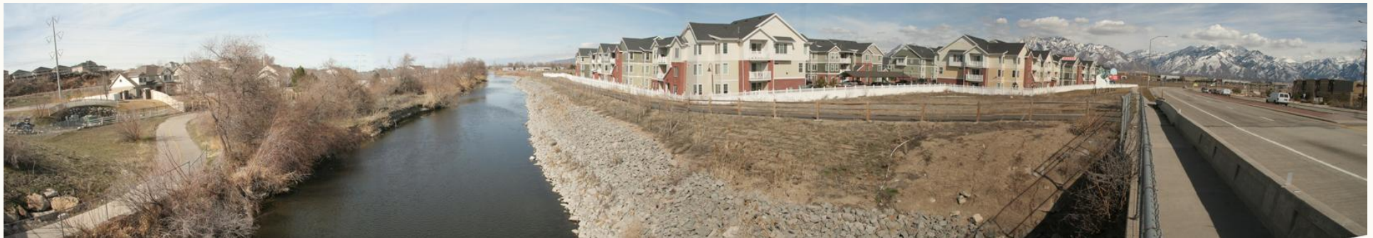
Typical business as usual worst practice Jordan River floodplain encroachment, streambed channelization and fortification, Murray
