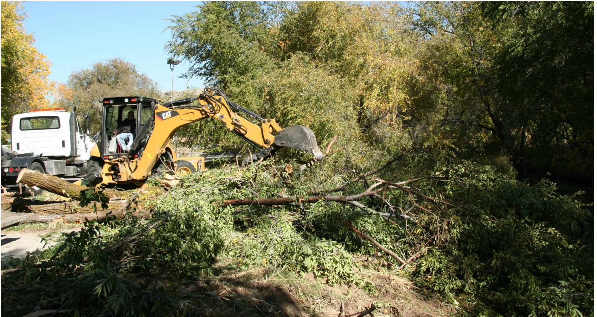
Typical Salt Lake County Flood Control streambank denudation project, Salt Lake City, October 2008. Access for large equipment typically requires the removal of whole groves of trees.
