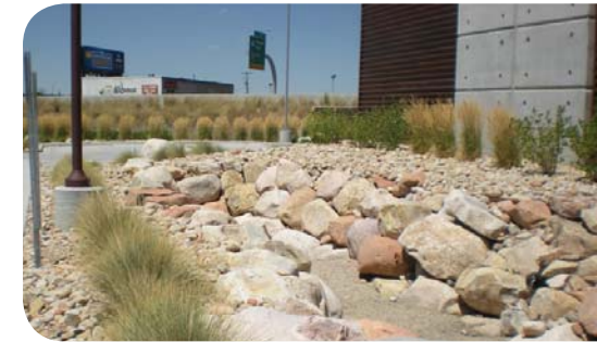
Local Project Success: ACG Building, West Valley City Stormwater detention landscape Photograph by Nancy Monteith
