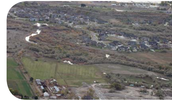
Local Project Success: Springview Farms, 146000 South, Bluffdale Photograph by Chris McCandless
