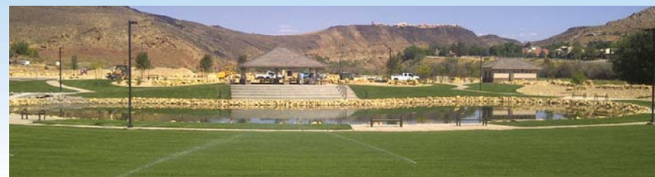
Washington Fields Detention Basin, Washington, Utah (Courtesy: URS)
