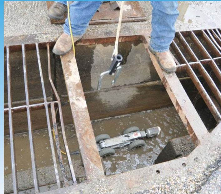
Camera inspection of a stormwater facility Source: blog.udot.utah.gov
